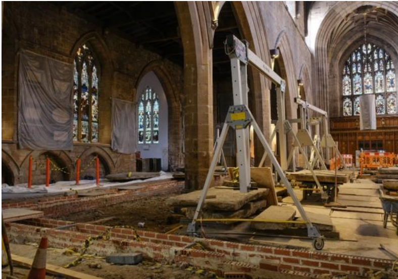
Brick conduits for the services with lifting A Frames
