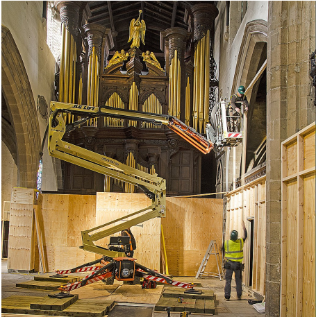
(L) Bump protection and segregation for dust control.
