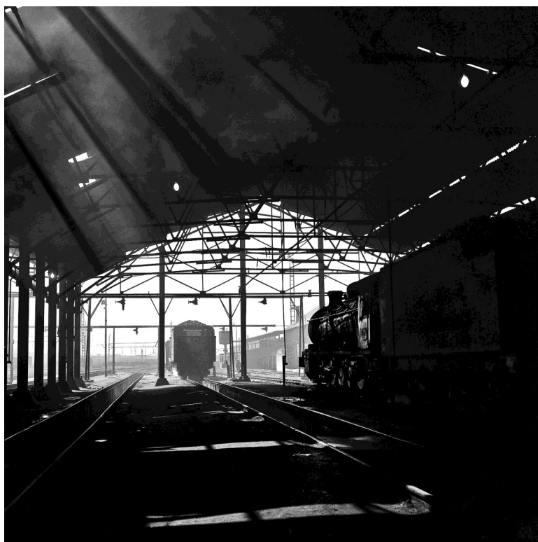
Inside the loco sheds at Germiston
